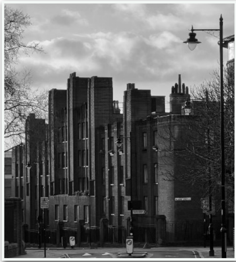
Charles Rowan House before the renovation began.
