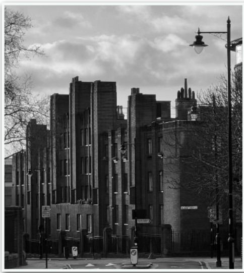
Charles Rowan House before the renovation began.
